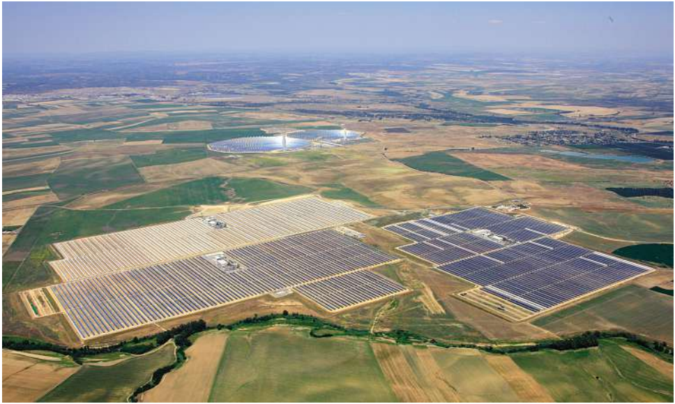
Fig. 4 Parabolic solar power plants Solnova 1, 3 and 4 (3 x 50 MW el ) in San Lucar near Seville. In the upper part of the picture there are the two solar tower power plants PS 10 and PS 20 with a capacity of 10 respectively 20 MW. [Source: Wikipedia]
